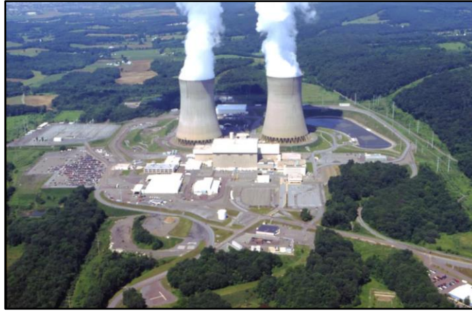
Susquehanna Nuclear Power Plant
